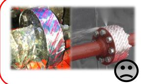
Convenient tape solution, should be wrapped with 50% overlap, all the way down to pipe.
