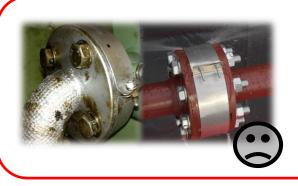
Held tight against the flange, generally with poor connection design with open gaps.
